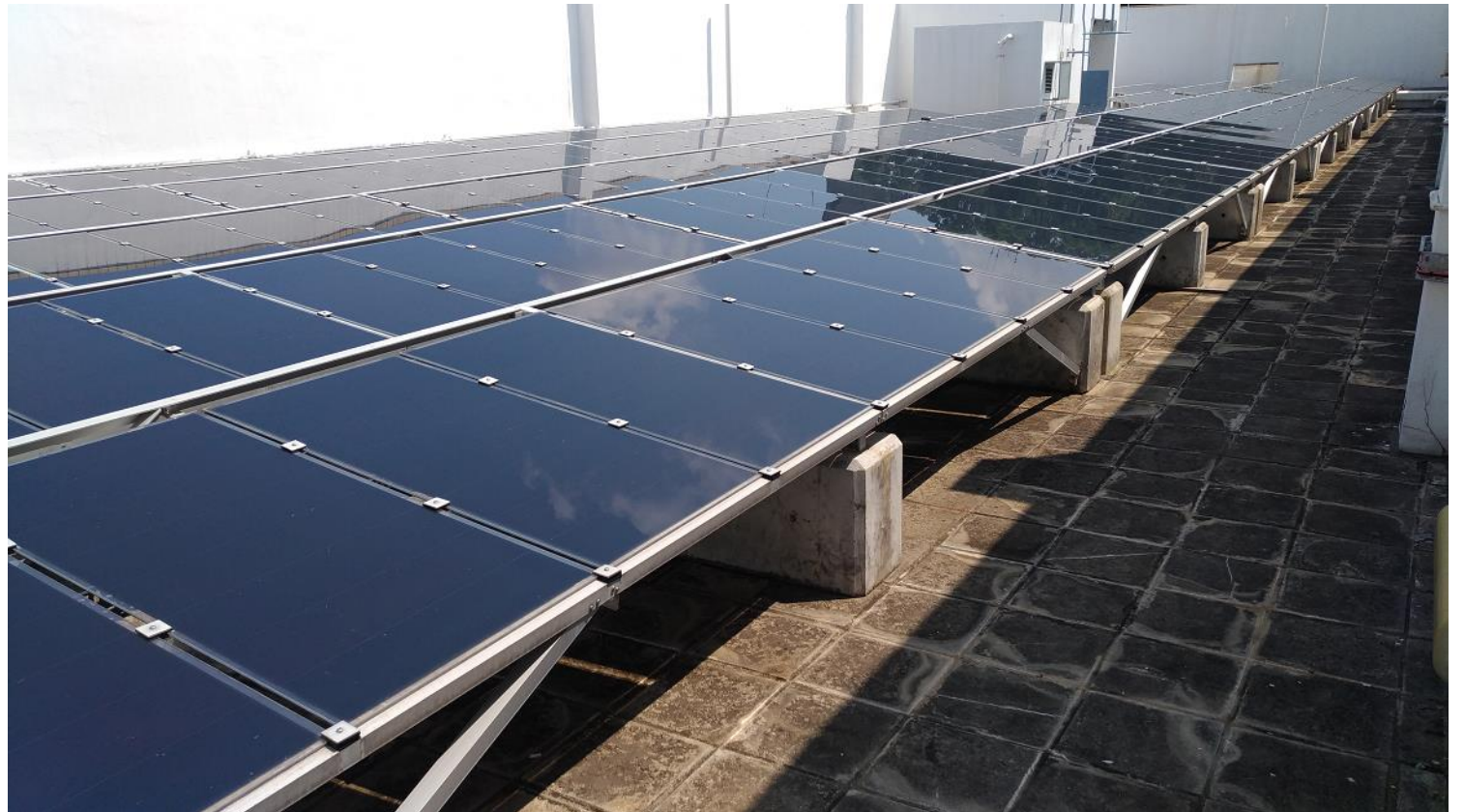
CUHK 37kW On Grid System
