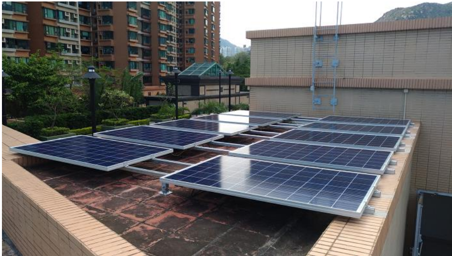
Household, N.T. 2.5kW On Grid System
