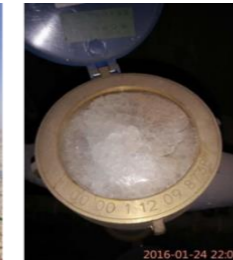
Frozen Water Meters & Pipes
